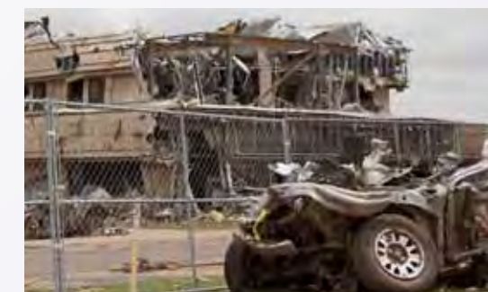
An Oklahoma shopping center after the 2013 tornado.
