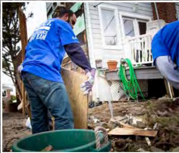
IRUSA volunteers help with cleaning and repair efforts in New Jersey after Hurricane Sandy.
